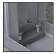
Fasten anchors to floor with specified washers.
